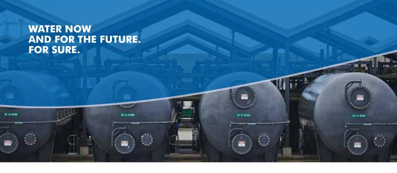
The Victorian Desalination Project uses a two pass reverse osmosis process to remove minerals and salts and produce a product that meets strict water quality requirements.
