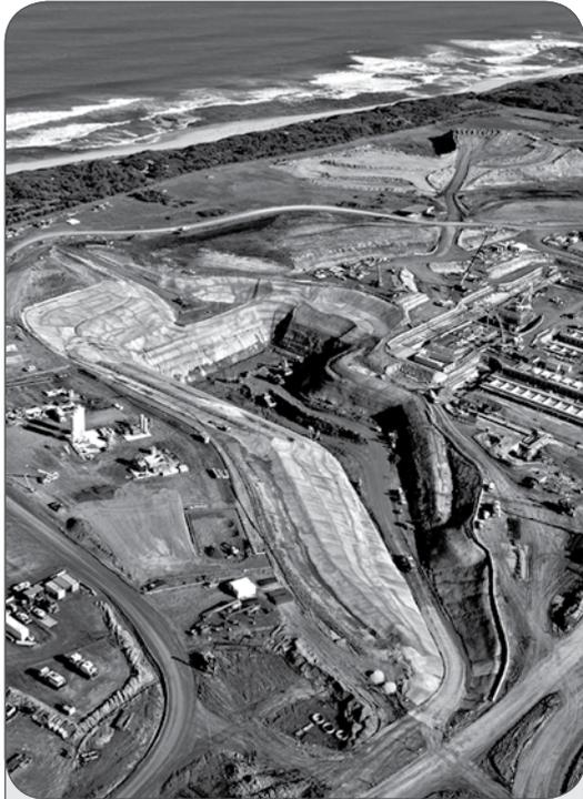
The box cut is nearing completion, ready for tunnelling
