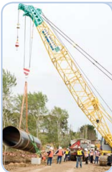
Pipeline: A crane lifts a pipe into place above the trench
