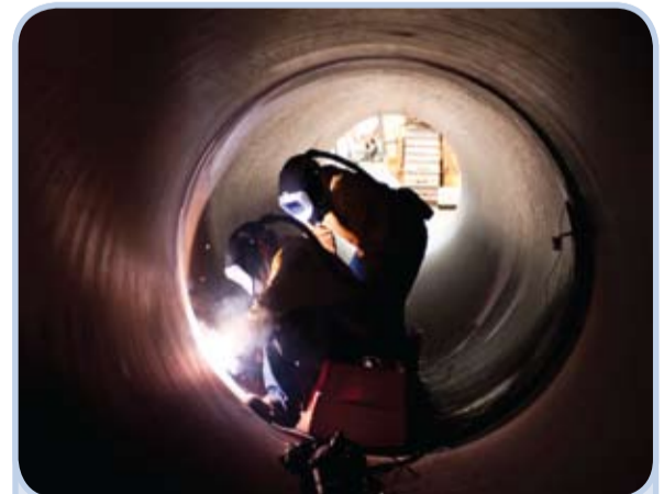
Pipeline: Pipe sections are welded together
